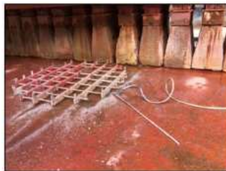
Thruster grating being cleaned at the time
