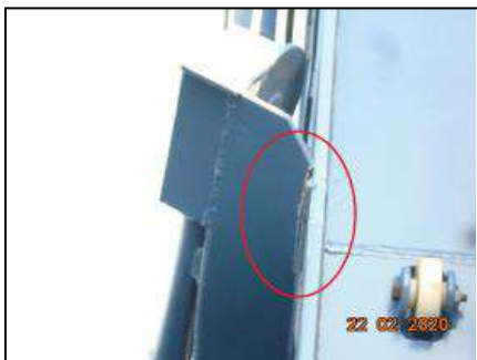
Cracked welding
