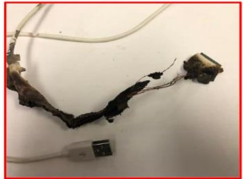
Wire insulation apparently failed, leading to fire.
