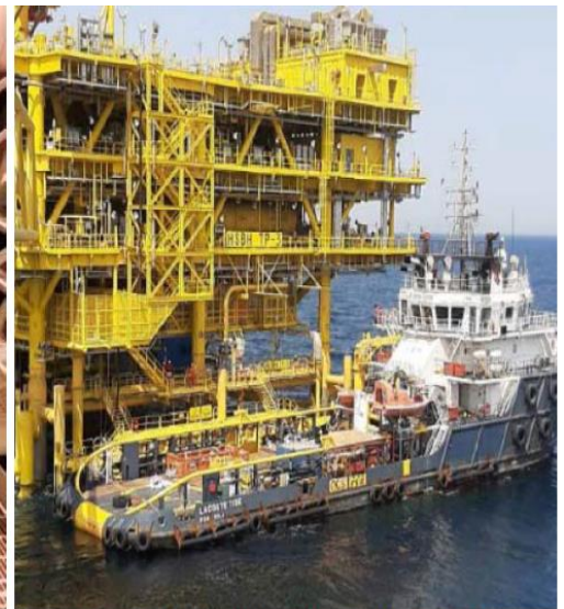
Offshore platform where incident occurred, with workboat alongside (moored to boat-landing)
