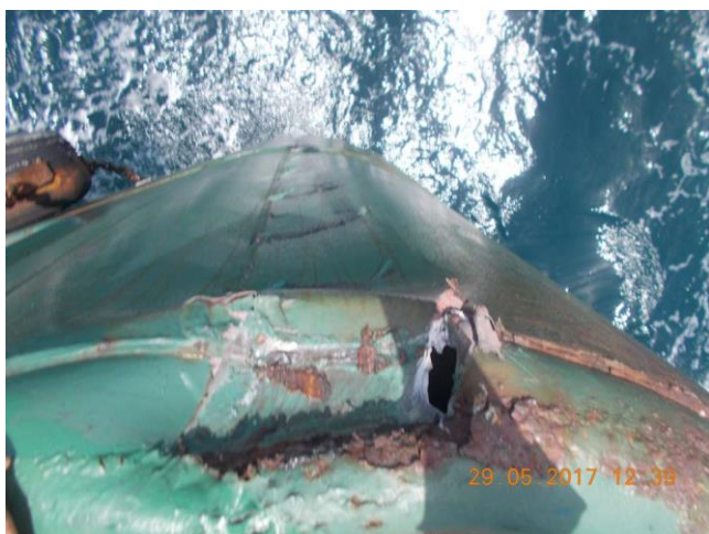
Dent in PSV as a result of collision
