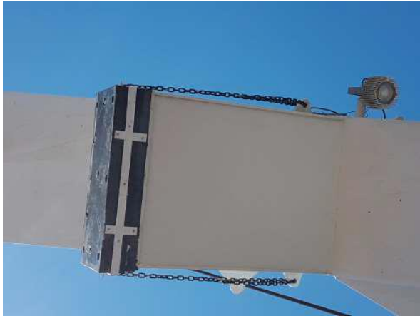
Showing buffer plate and subsequent secondary securing chains
