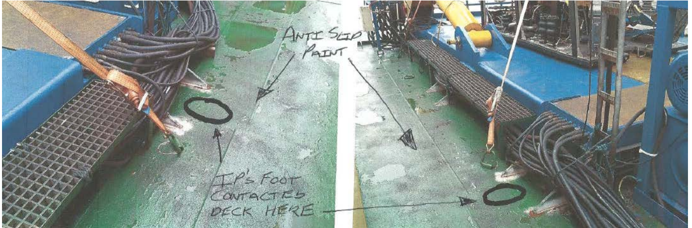
Showing worksite where injury occurred
