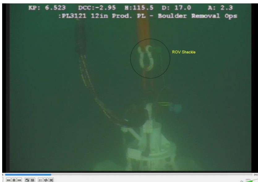
Showing shackle (white) and pin (green) partially disengaged.
