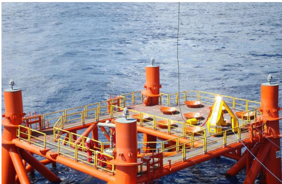
Jacket showing personnel transfer capsule and crane wire
