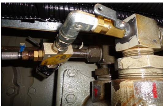
Connection after initial temporary repair
