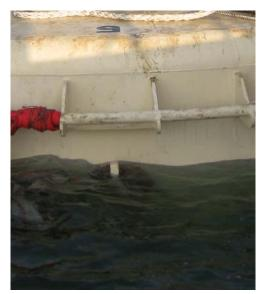
Sling Preparation 4m\*6mm 4m\*6mm Duck Tape Step 3 Step 2 Step 1 Secure one eve on the Pass the hook by typing the 6mm rope to the fender Tie the second Dyneema Sling 6mm rope to through the the fender to masterlink keep the eye on the hook and back on to the hook The diver can then stand clear and observe while the crane is lowered until the weight is transferred from the crane to the Dyneema Sling
