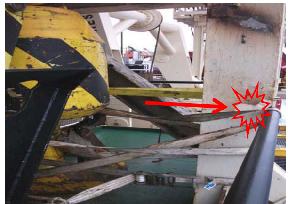
Crane block and upright showing how crane block moved
