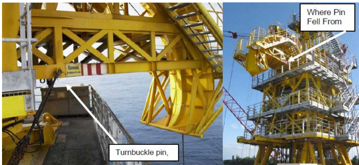
Location of turnbuckle pin (L) and where the turnbuckle pin fell from (R)
