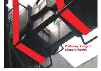
Figure: Showing re-assessed lifting point arrangement used after incident
