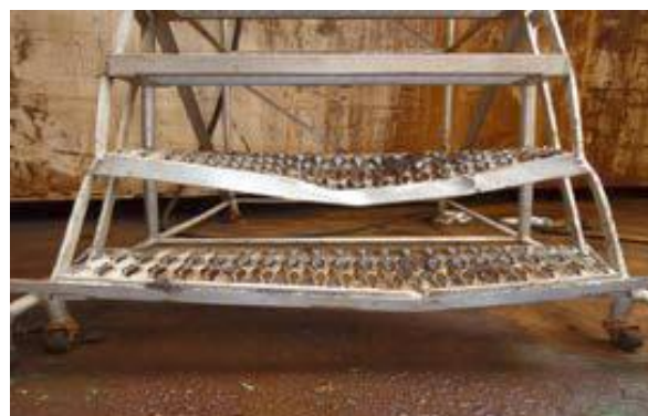
Figure 2: Showing damaged steps
