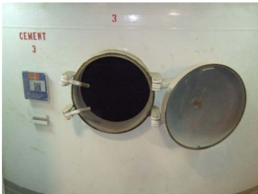
Cement tank hatch
