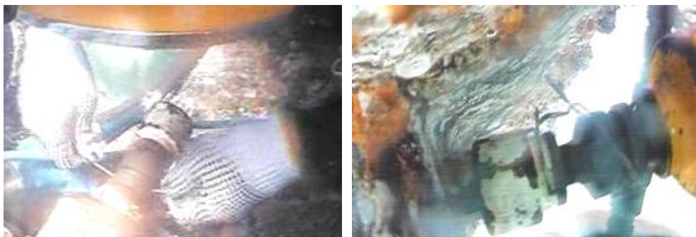
Showing use of welding rod as a retaining pin
