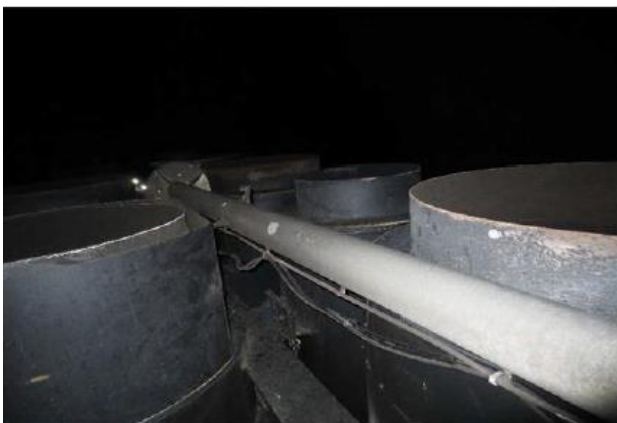
Mast resting between the stacks
