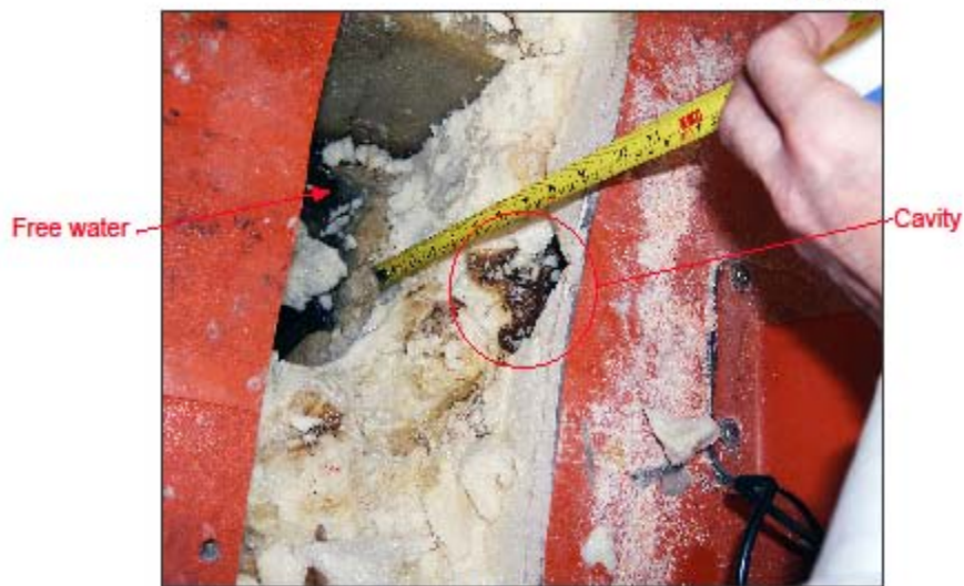
Below deck inspection
