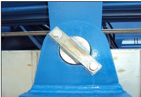
Lift post pin installed.
