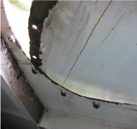
Inspection hatch being prepared
