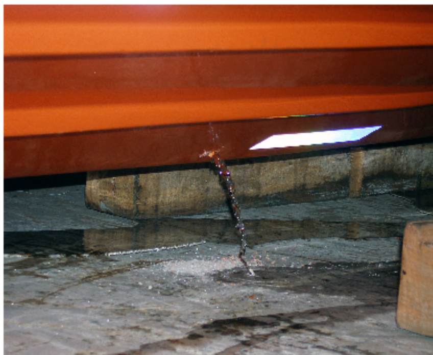
Water draining from foam-filled compartments
