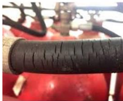
Brittle hose on fixed CO 2 bottles
