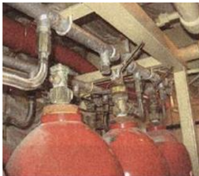
Disconnected CO 2 bottles
