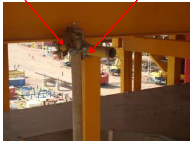
Showing details of scaffolding
