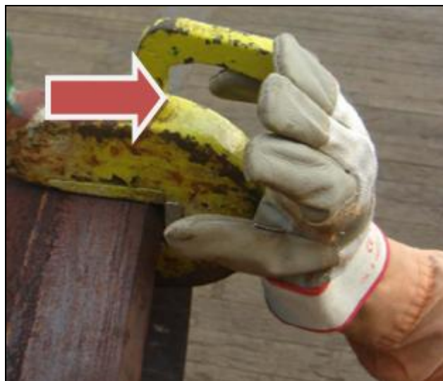
Illustration of right hand position holding the pipe hook
