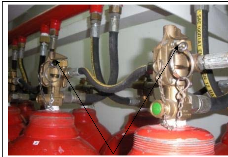
Safety pins in position. These MUST be removed for the system to function
