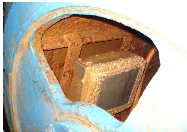
Opening into drum and rotary junction box
