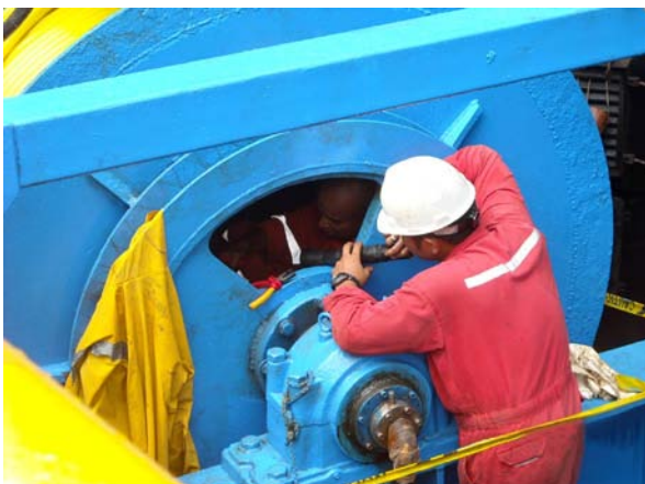
Umbilical winch drum and small opening
