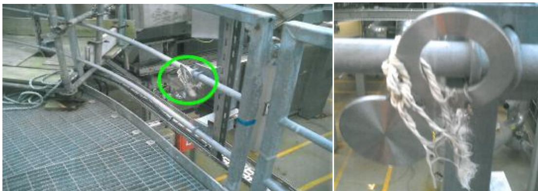
Showing spade secured to handrail
