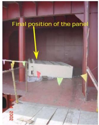
After 3m transfer into the room, the panel bottom lost contact with one of the rollers, becoming destabilised. The panel toppled over and trapped one of the workers. He was crushed and died instantly.
