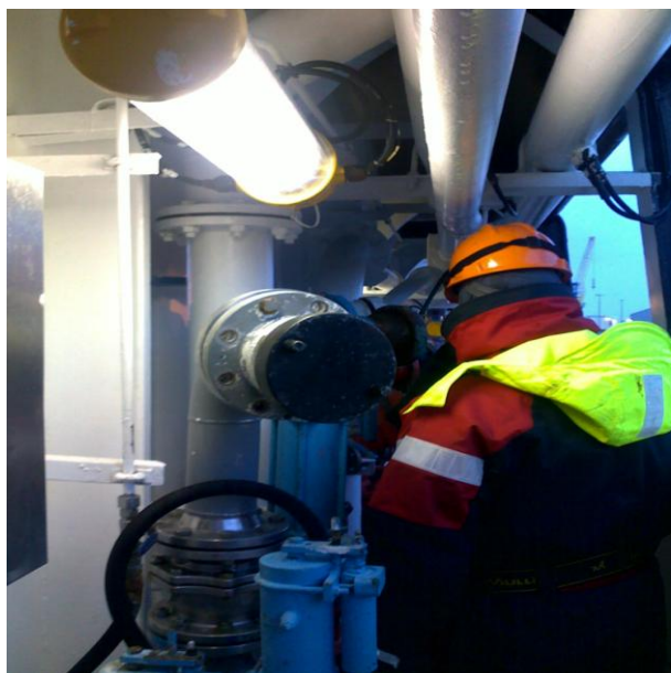
Showing discharge manifold from which cap was blown
